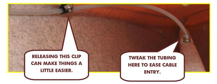
Feed the cable in carefully as I found that getting it around the 1<sup>st</sup> bend was a little awkward. Overcome this by just tweaking the tube a little. You find it easier still if you undo and release the retaining clip. Continue feeding in. If you are lucky the new cable will run right the way through. If, like me, it doesn't then you'll probably find that the cable has stopped at the point where it is supposed to enter steel slider tube.
