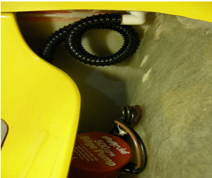
pump not wired up yet
